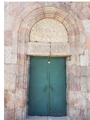
Fig. 2. Use of single-stone lintel in Emir Saltuk Cupola, Erzurum-Turkey
