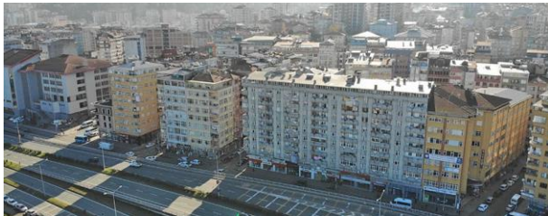
Fig. 2. Buildings to be Demolished within the Scope of Rize Urban Renewal Project Stage 1
