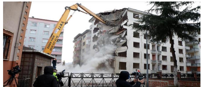
Fig. 4. Rize Urban Renewal Project 1st Stage Demolition
