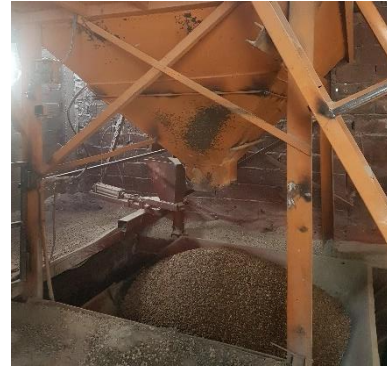
Fig. 4. Pumice aggregate in bunker just before mixing
