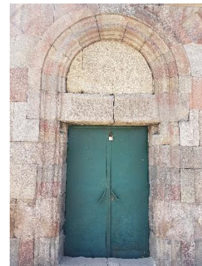
Fig. 2. Use of single-stone lintel in Emir Saltuk Cupola, Erzurum-Turkey
