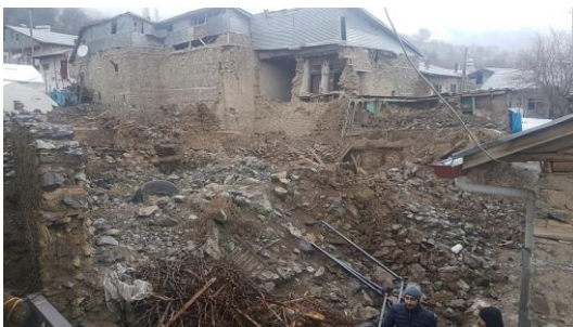
Fig. 5. Total Collapse of Adobe Structures in Sivrice Earthquake - Duygulu Village – Courtesy of Dilek Okuyucu
