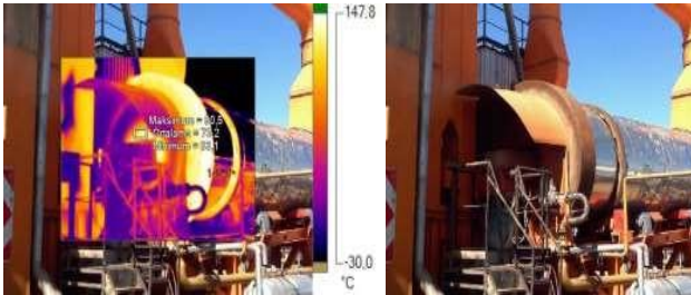
Figure 4. Surface thermal imaging of drying unit.
