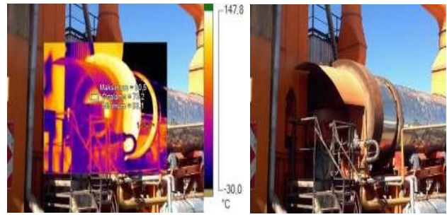
Figure 6. Surface thermal imaging of drying unit.
